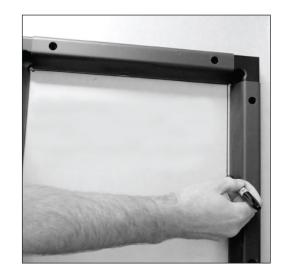
(A)Position frame on cabinet base; clear of obstructions below. Outline the frame's inside edge for cutting.
